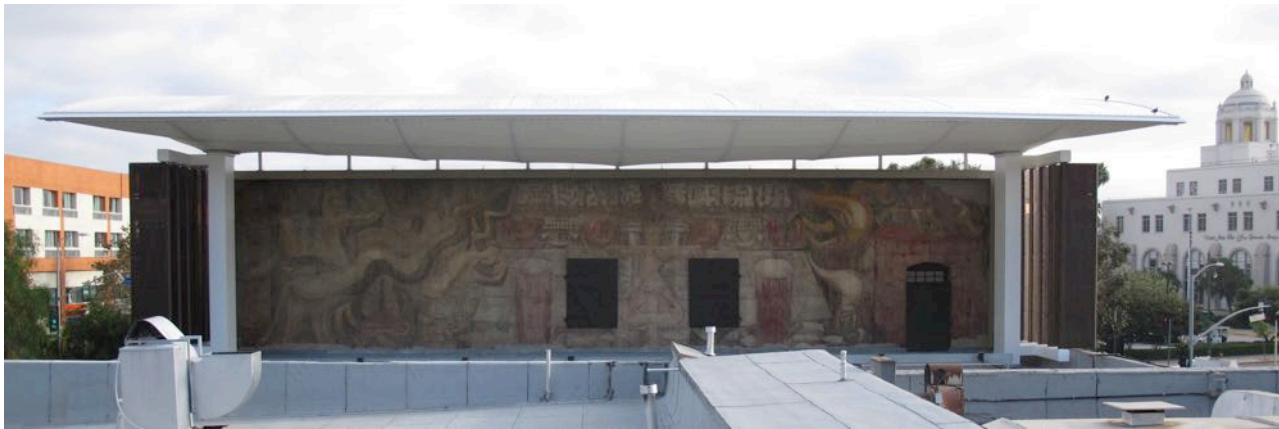
Image caption: América Tropical, David Alfaro Siqueiros, 1932, after conservation treatment and construction of a protective canopy shelter. Photo © J. Paul Getty Trust, 2012. Mural © 2020 Artists Rights Society (ARS), New York / SOMAAP, Mexico City.
